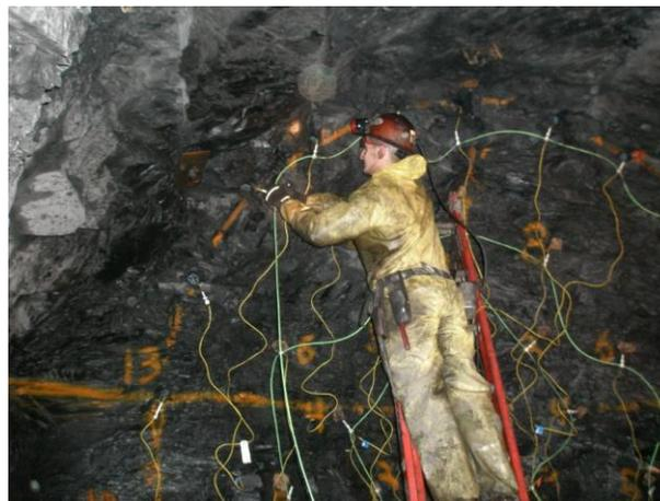
*Figure 7 – Tying up at heading*
